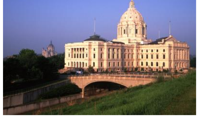
Minnesota State Capitol Building.
